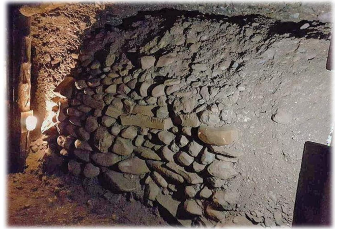
Figure 6. Dry-stone wall constructed within a Ravne tunnel passage, forming a structural barrier that restricts access to adjacent sections.
