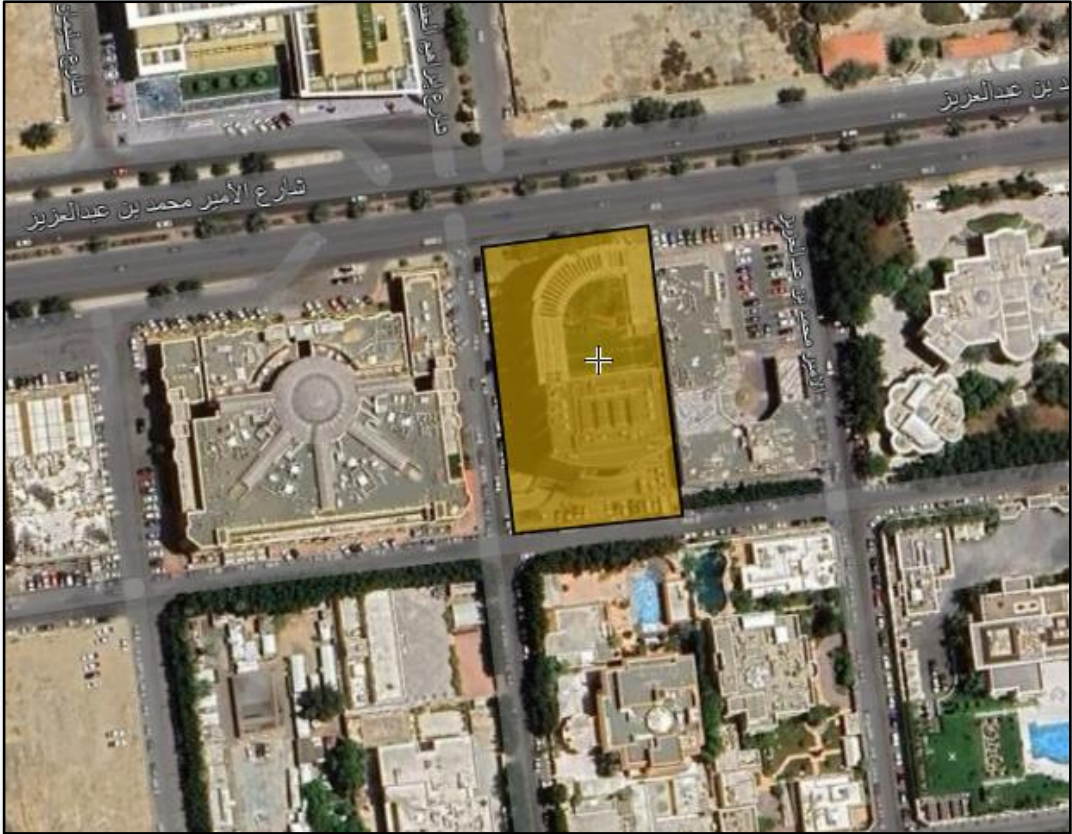
Property located at Neighborhood level
