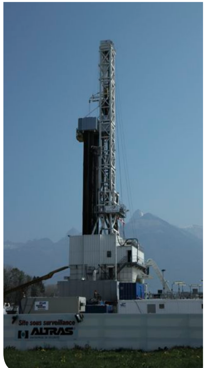
Drilling for hydrocarbon prospection in Noville (VD, Switzerland).
