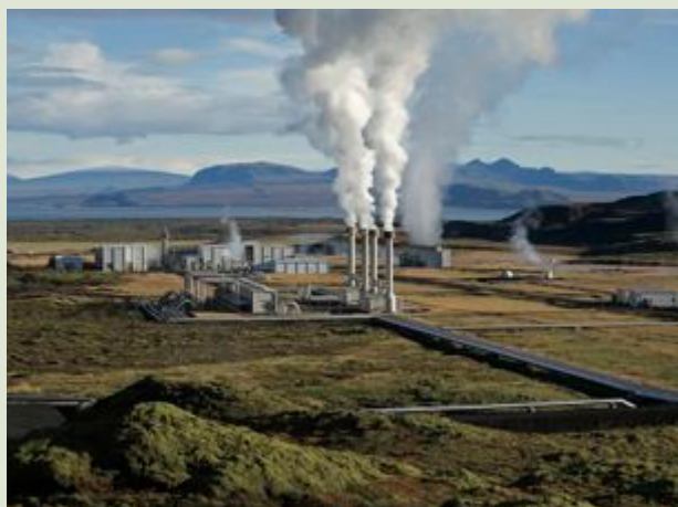
Geothermal power plant in Iceland.
